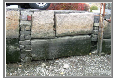
PHOTO 8 A&B Mechanic St Seawall – note unusual vertical joint construction
