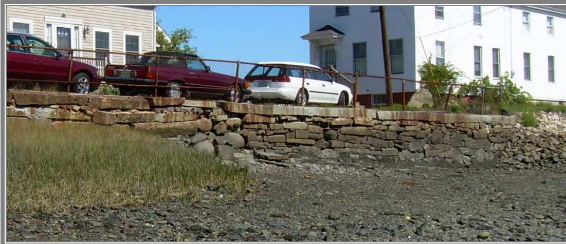
PHOTO 5 South Mill St Seawall eastern end.
