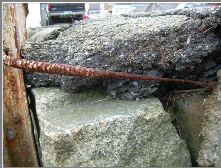
PHOTO 9 Mechanic St Seawall – severely corroded tie-rods
