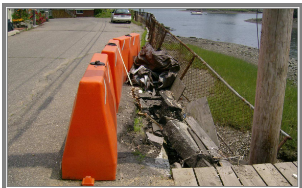
PHOTO 3 (left) South Mill St Seawall looking west – note wall leaning offshore.
