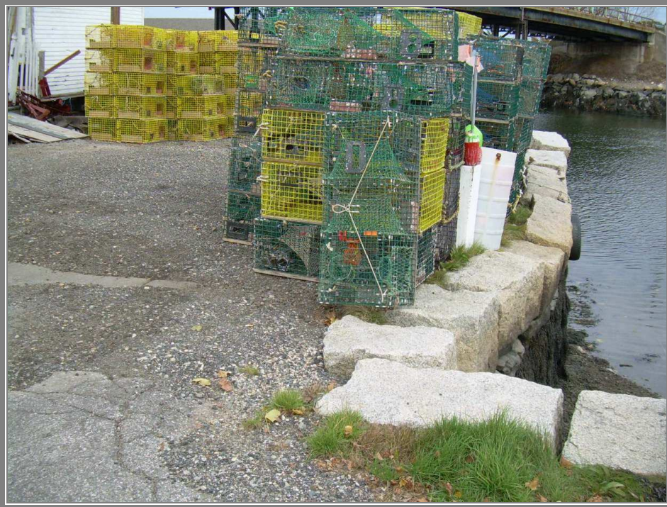
PHOTO 12 Mechanic St Pump Sta. Seawall – perpendicular wall with pronounced bulge.
