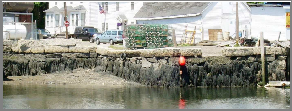
PHOTO 10 Mechanic St Pump Sta. Seawall – note missing cap stone to the right of the orange buoy – outfall is to the left of the orange buoy.
