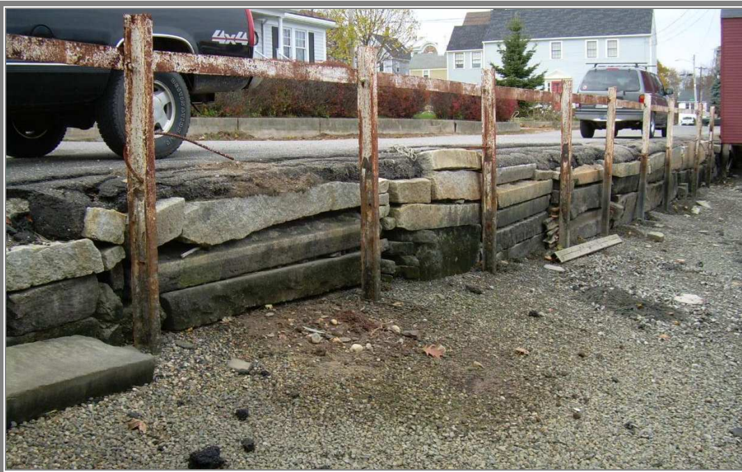
PHOTO 7 Mechanic St Seawall.
