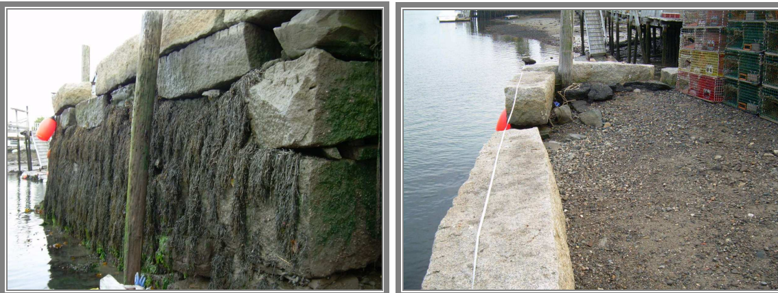
PHOTO 11 A&B Mechanic St Pump Sta. Seawall – outer wall.
