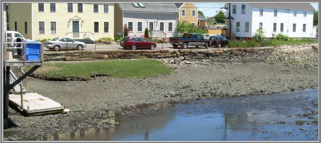
PHOTO 1 Overall view of South Mill St Seawall.
