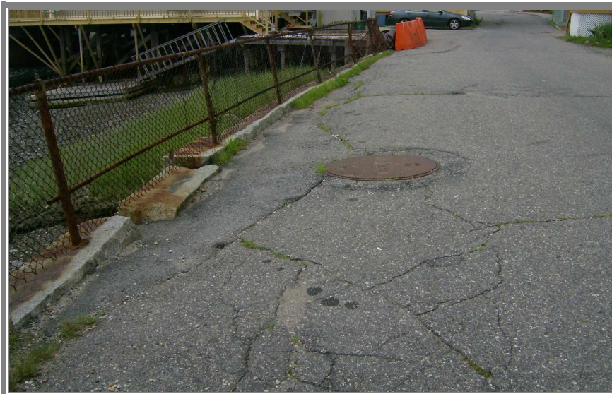
PHOTO 6 South Mill St Seawall – note sewer manhole close to wall.
