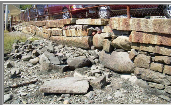
PHOTO 3 (left) South Mill St Seawall looking west – note wall leaning offshore.
