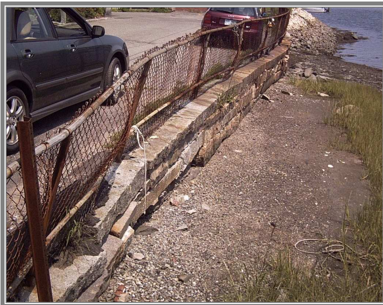
PHOTO 2 South Mill St Seawall looking east – note wall bulge and lean offshore.
